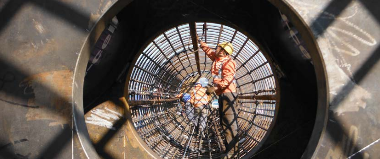
Installation of instruments for Osterberg Cell load test, Lantau, Hong Kong.
